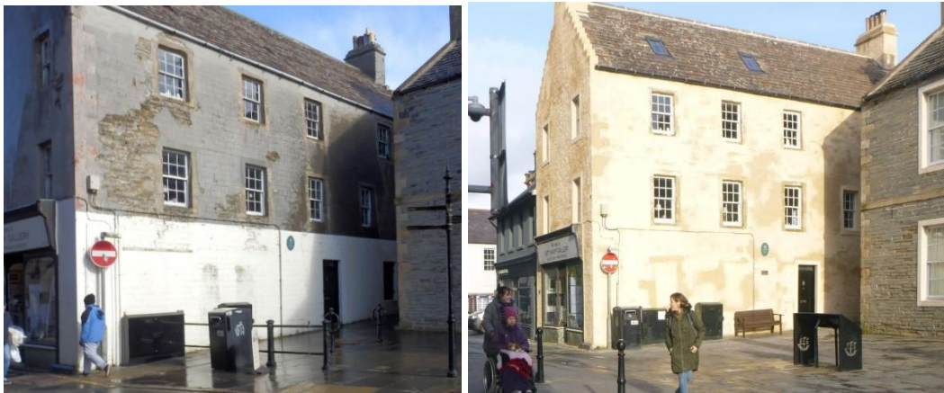
Above – Albert Street, property restoration
