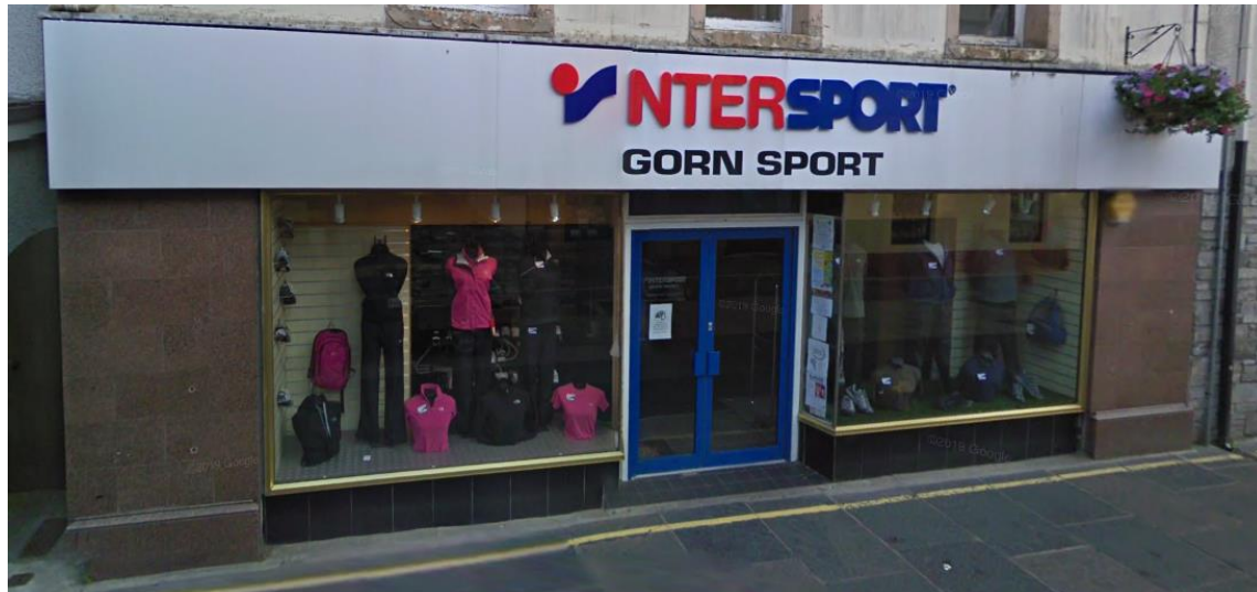
Shop front before works
