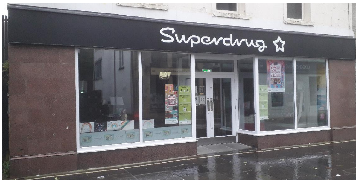
Shop front reinstated
