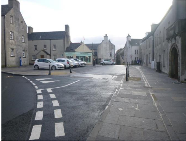
Above – the Victoria Street Gateway improvements with widened pavement enhanced public realm space enabled by reconfigured parking.
