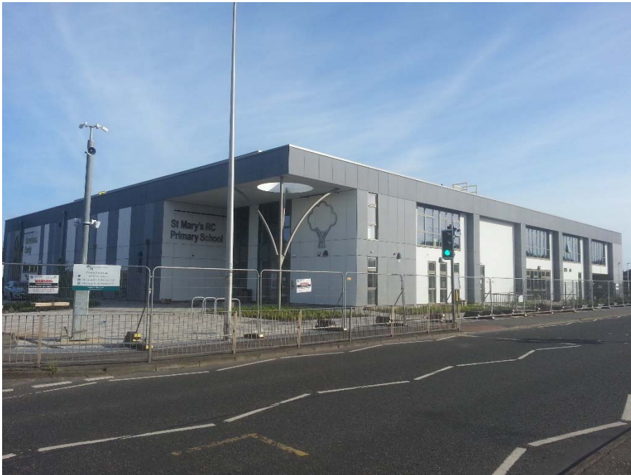
Construction at the new St Mary's/Burnbrae Primary School.
