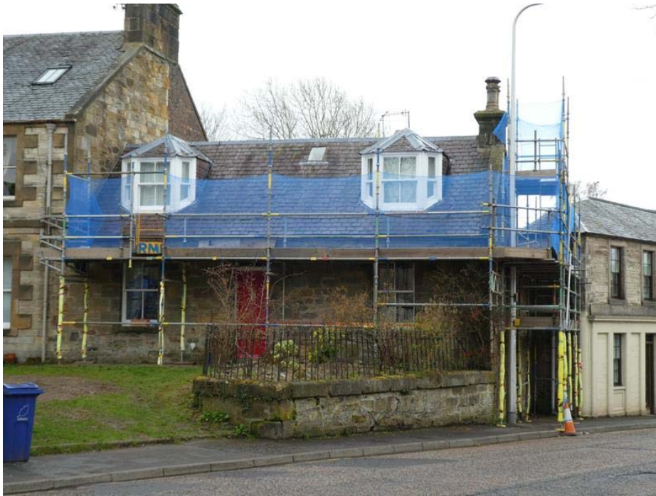
Restoration and repair work starting at no. 10 The Square.
