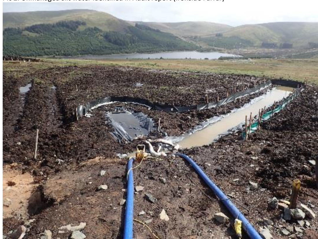
Pic 3. Polysorb pumping to remedy fuel spill at Turbine 15
