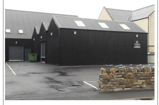
The scale relates to neighbouring buildings, and is based on a main gabled section, with the roof line continuing to the rear, but with a different cladding material to emphasise the traditional gable shape. A through-coloured fibre sheeting was used to clad the walls, with extensive glazing, dark framed windows and doors, and a black corrugated metal roof. Storage building to the rear were also clad on walls and roof with the same corrugated metal, echoing the former industrial use of the site.
