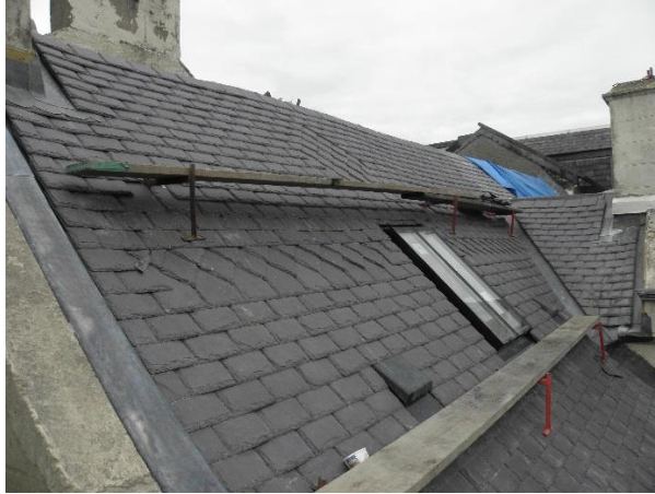
33-35 Bridge Street, Galston:- Complete reslating and rot repairs to the roof structure. To be completed August 2016.
